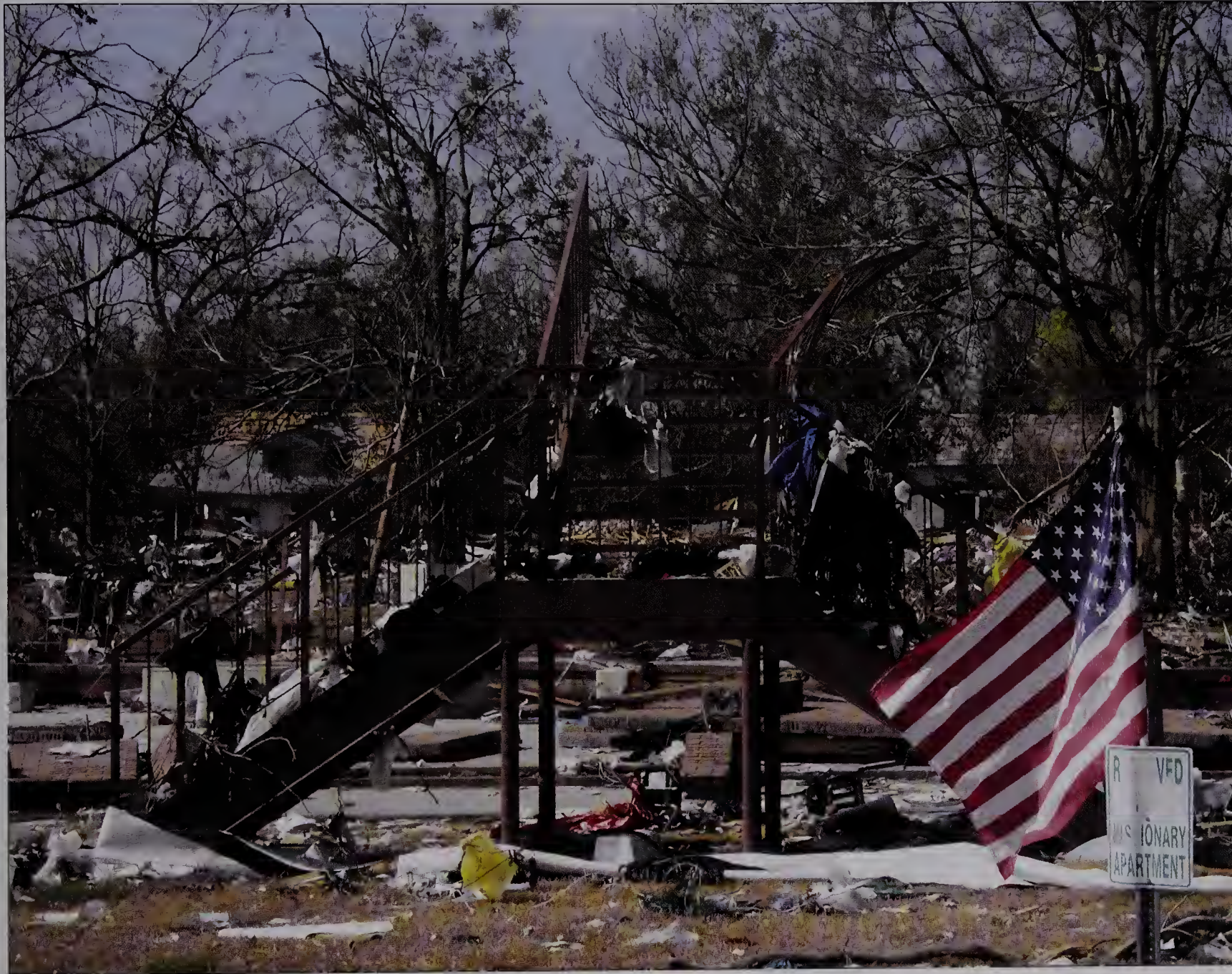
Ruins of apartment building, Long Beach, MS Denton Herring photo
